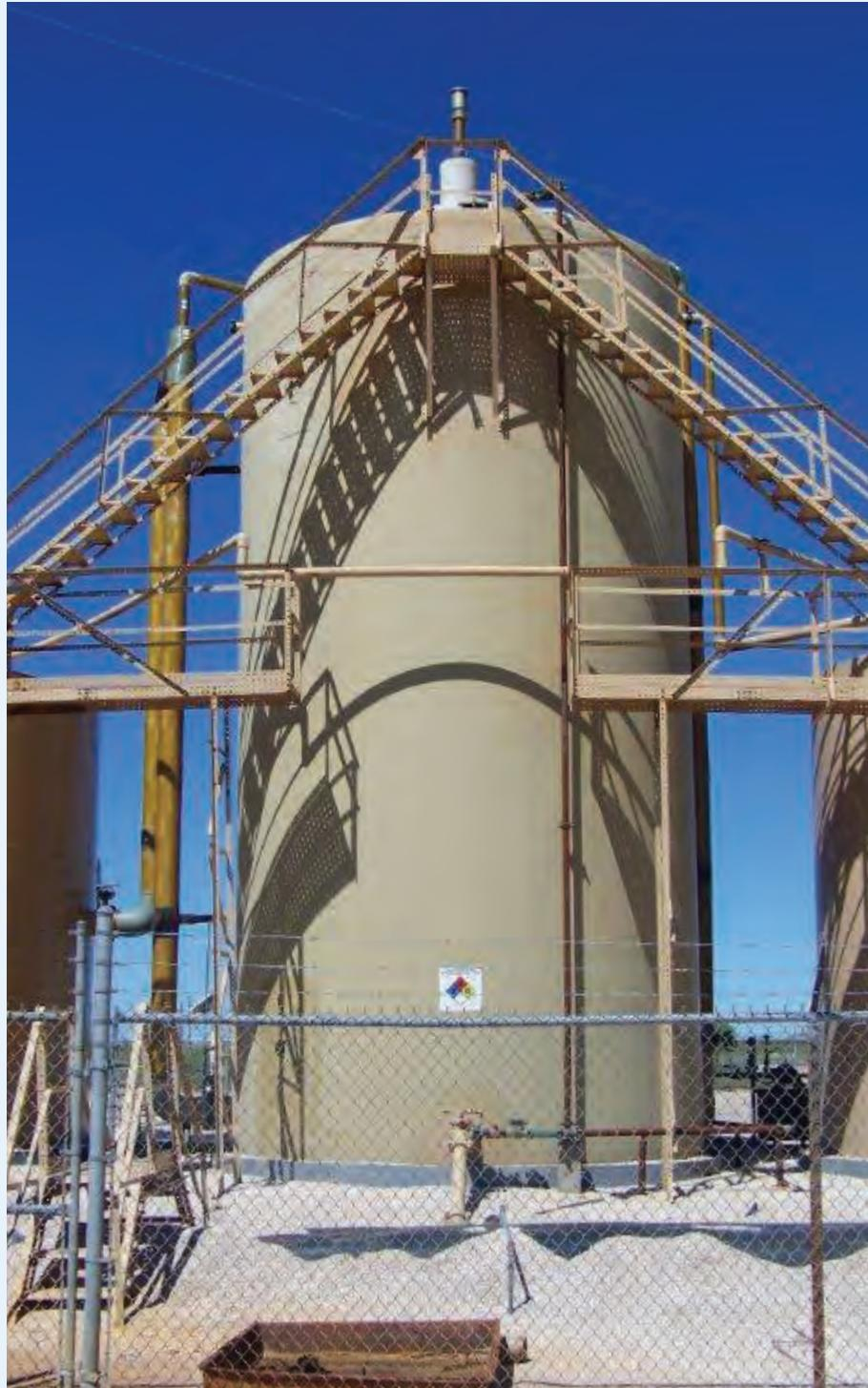
The gunbarrel is an economical and low maintenance method to treat oil when properly applied.
